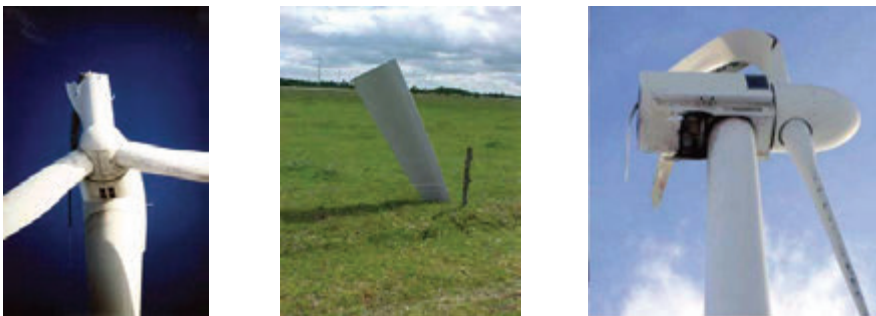
Figure 10: Damages due to defective rotor blades
